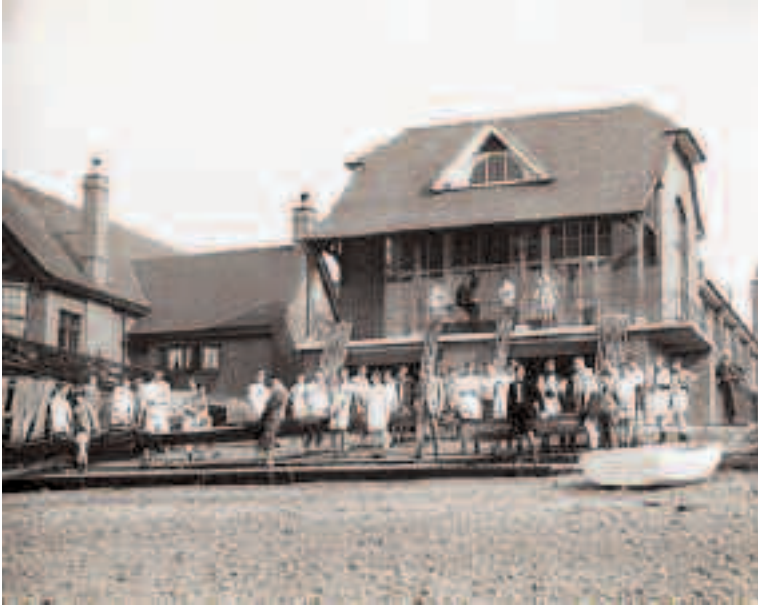
The boathouse after rebuilding in 1951.
